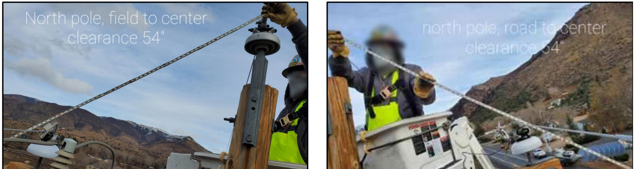
Figure 2: Annotated Demonstration of Measured Radial and Calculated Horizontal and Vertical Conductor Clearances
